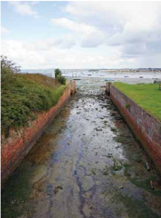
Milton Locks. This sea basin allowed canal boats access from the canal to and from Langstone Harbour when the tide was high. To supply the water for the rest of the canal, a nearby pumphouse drew water from a well and (at high tide) the sea.
